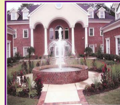
LCW is located in the South DeKalb Business Park on Wesley Chapel Road
